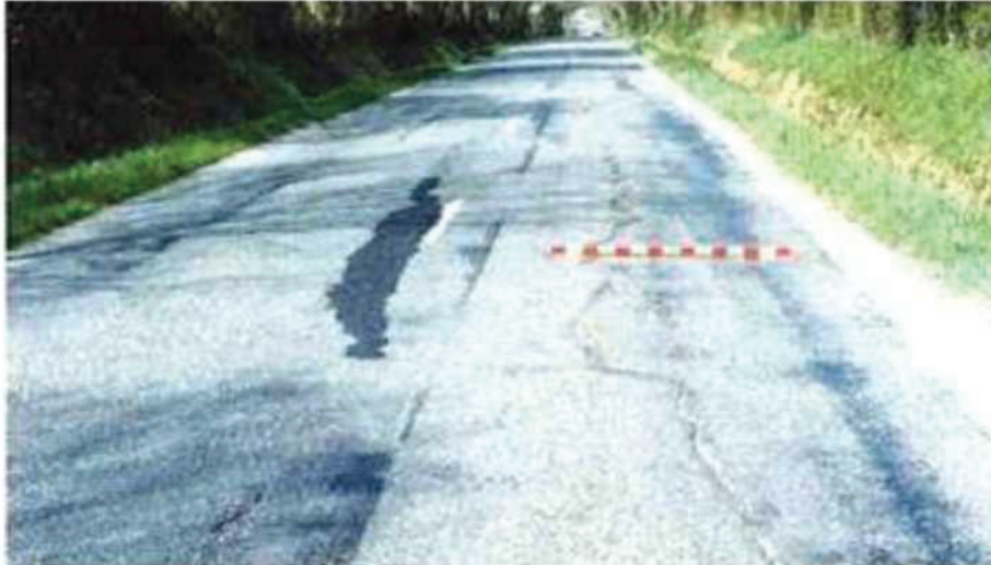
fig.II.6 : fissuration d'adaptation
