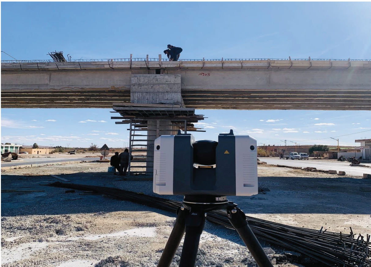
FIGURE II.5 : Le scanner laser leica RTC360
