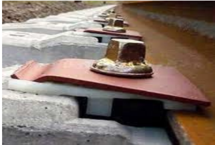
Figure III:5 Attache type Nabla
