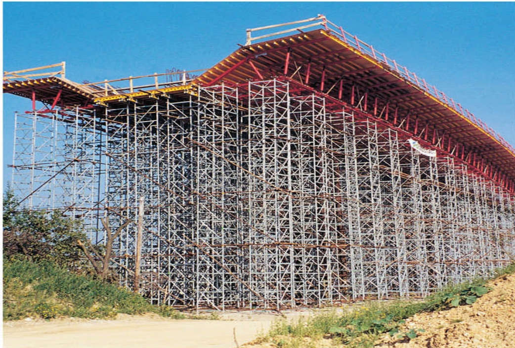
Figure 2. 21 : Coffrage type PERI
