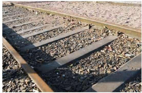
Figure III 7 Traverses métallique [5]
