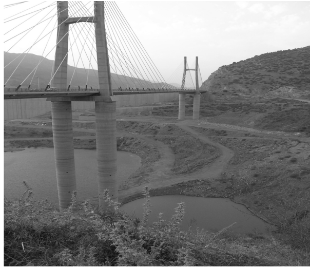
Fig. 2 General view of Mila's Cable Stayed Bridge
