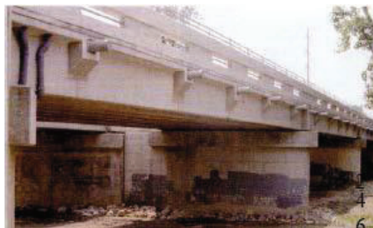
Figure I.4. Bridge Street Bridge Michigan (USA)
