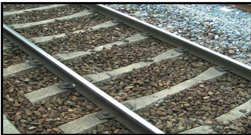
Figure III.5. Traverse monobloc.
