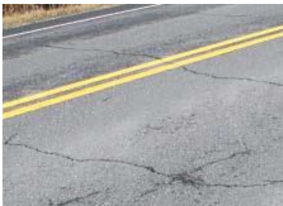
Figure I 1: Fissure transversale.
