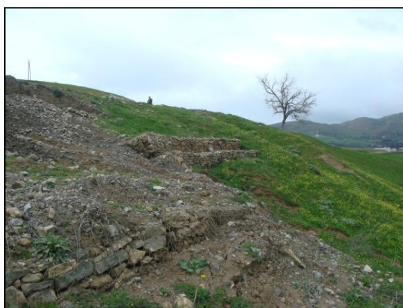
Figure II.6 : Gabions endommagés
