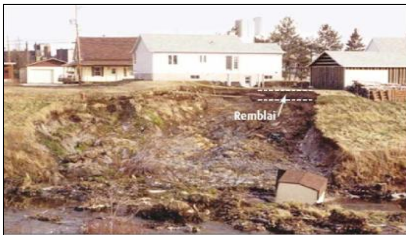
Figure I.9 :Construction sur pente
