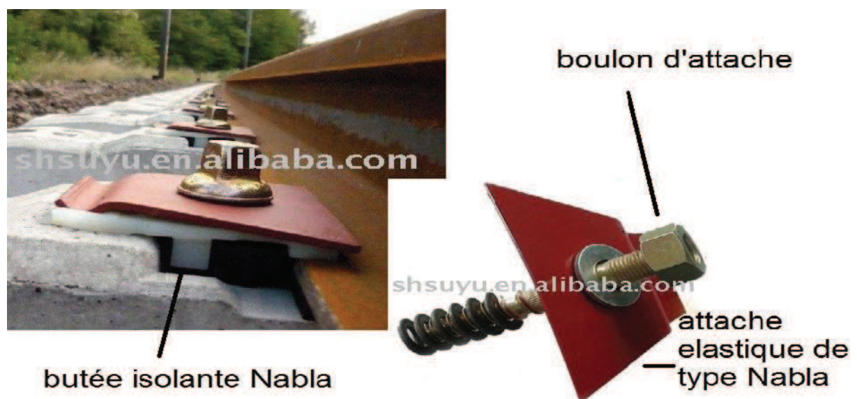
Fig.III.18: attache type Nabla
