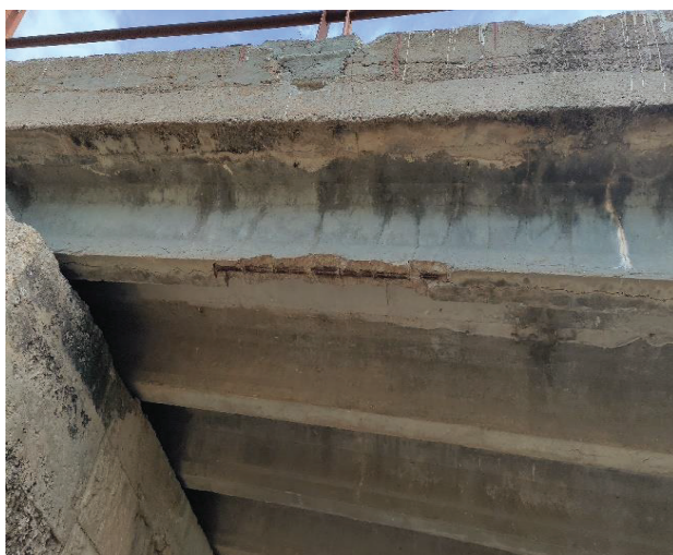
Figure X.4 Pont PK 77+850 – 6 X3.3m – Oued Enachef (A conforter la structure – Section hydraulique suffisante)
