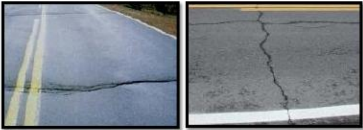
Fig.III.7: Fissures transversales.
