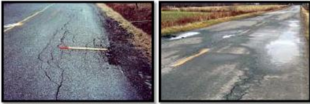
Fig.III.17: Affaissement
