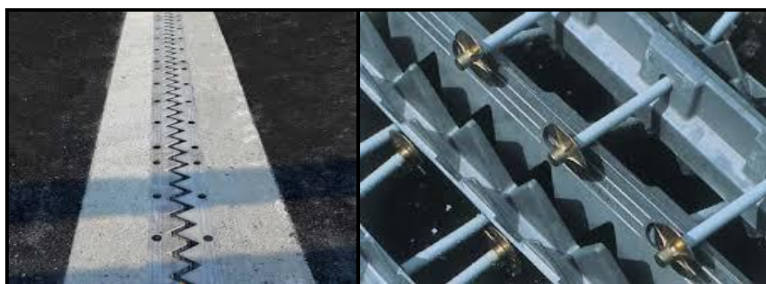
Figure XI. 10. Joint du type Wd80
