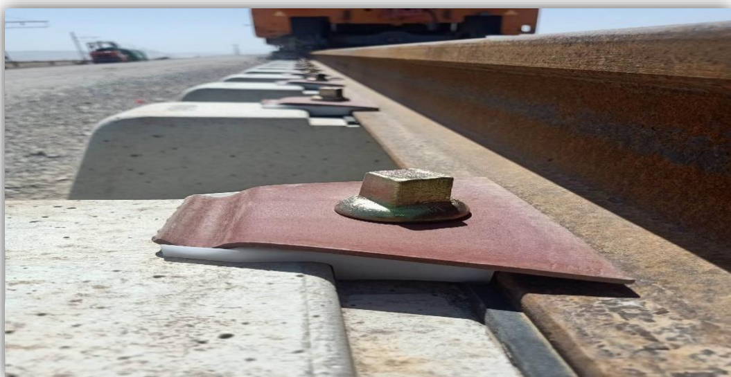
Figure III 5, Attache type nabla
