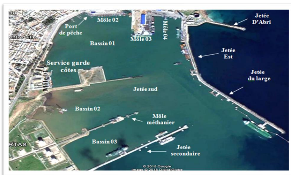
Figure II.2 – Infrastructures existante au Port d'Arzew
