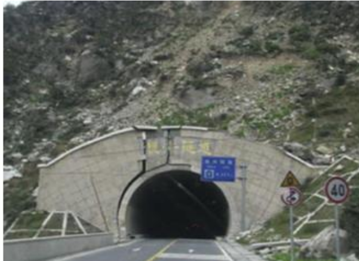
Figure I.9 : Classification des dommages sismiques (Shen et al., 2014)
