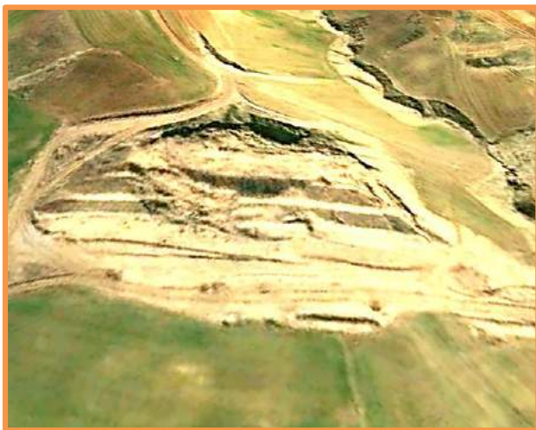
Figure 38: photo de glissement N 0 =2
