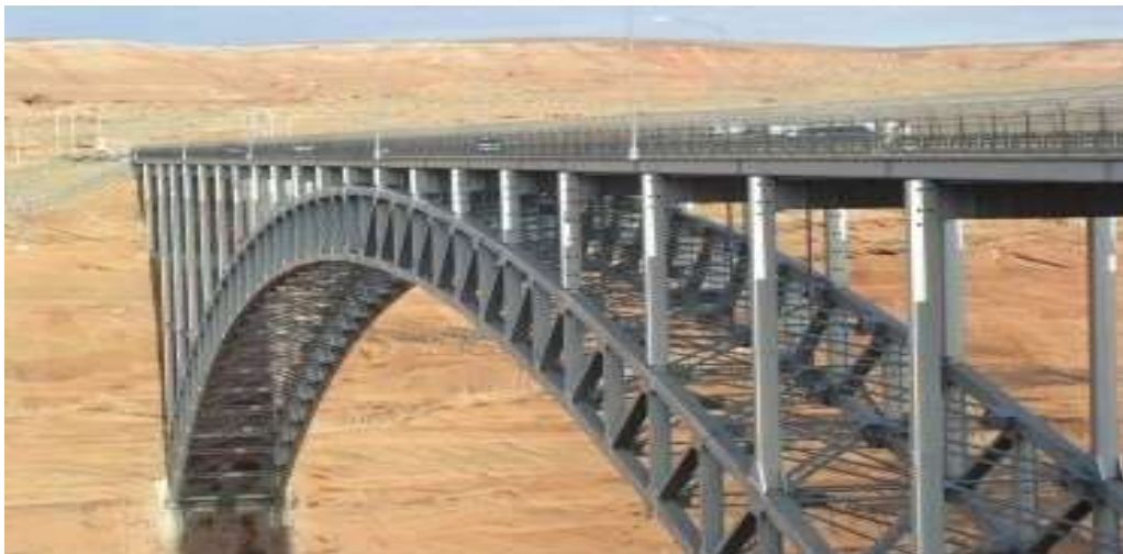
Figure I.9 : Le Glen canyon bridge
