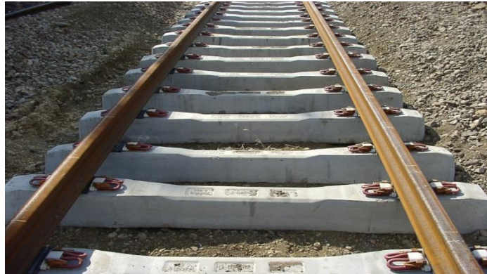
Figure I-2 Traverses monobloc
