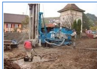
Figure 11 Sondeuse carottier [Source Google Image]
