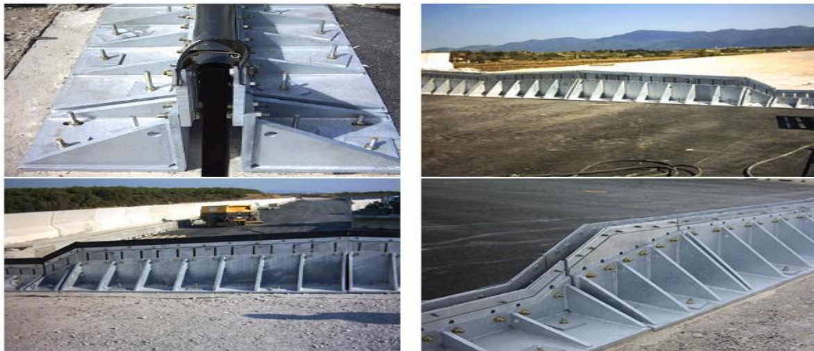
Figure IX. 5 : joint de ballast.
