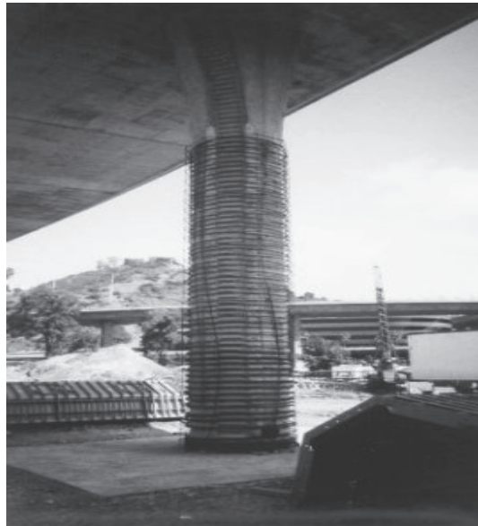
Figure I. 4 Renforcement du confinement.
