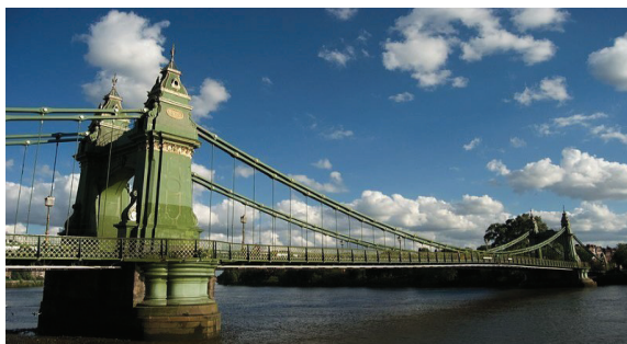
Figure II. 6 Pont de Hammersmith
