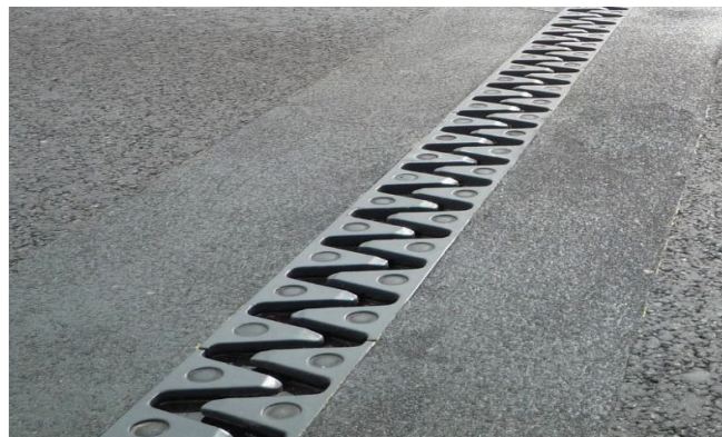
Figure VII.3. Joint de chaussée REJ100.
