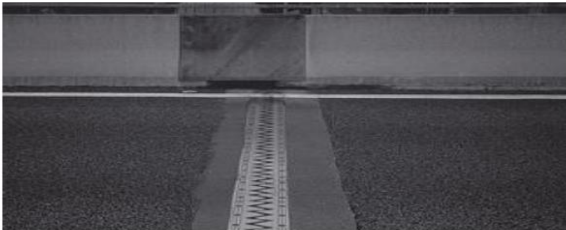
Figure VIII- 5 Joint de chaussée
