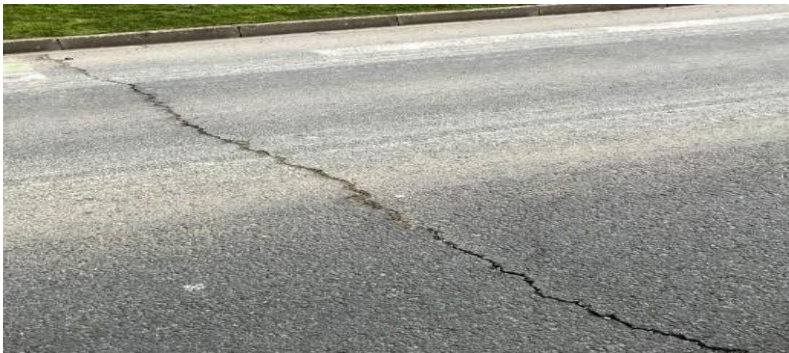
FIGURE 1 FISSURE TRANSVERSALE
