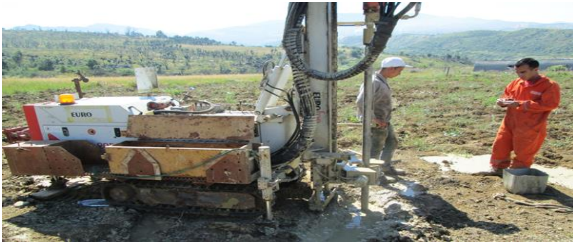
FIGURE 22 EXECUTION DU SONDAGE
