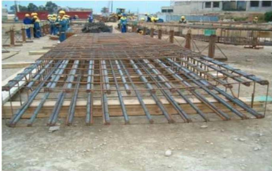
Figure V.4: cage d'armature
