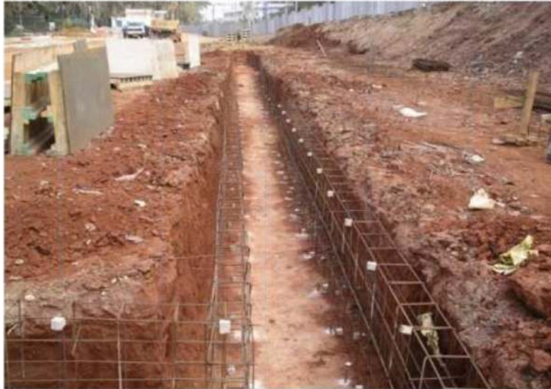
Figure V.5: tranchée guide
