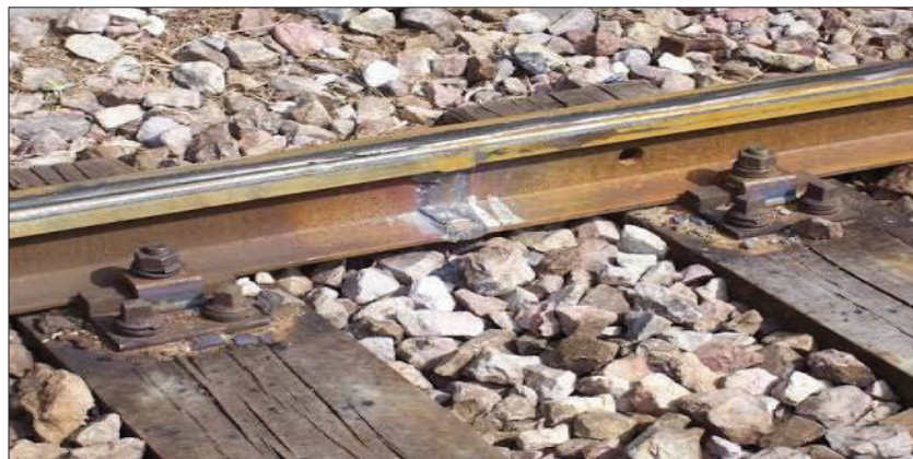
Figure IV. 4:Long rail soudé (LRS).
