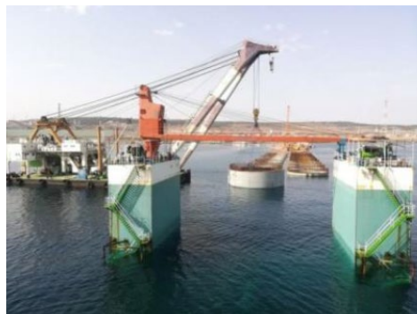
Figure II.24 : Installation du caisson
