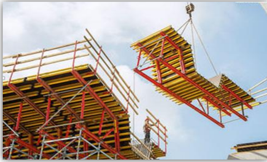
Figure III.21. Pose du coffrage.
