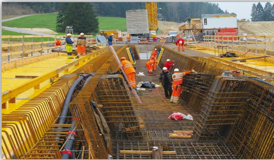
Figure III.22. Ferrailage du tablier.
