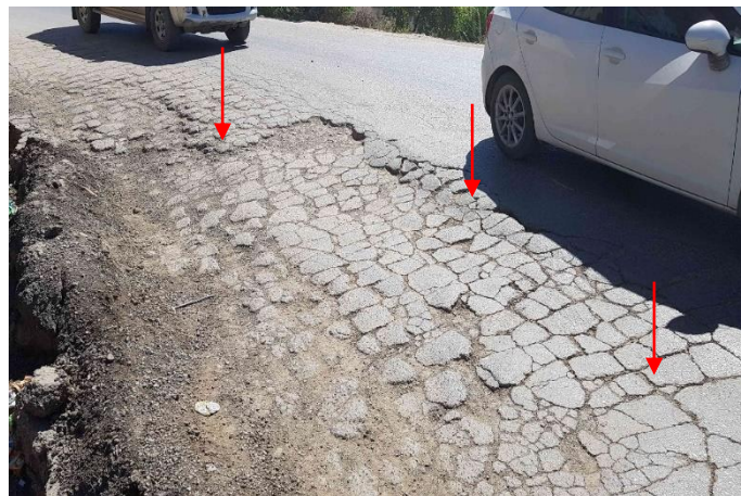
Figure III.11 Les tassements.
