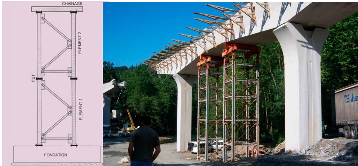
Figure III.11 : Palée provisoire
