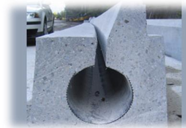
Figure 10.4: caniveau a fente
