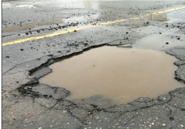
Figure I-8 : Nid-de-poule.
