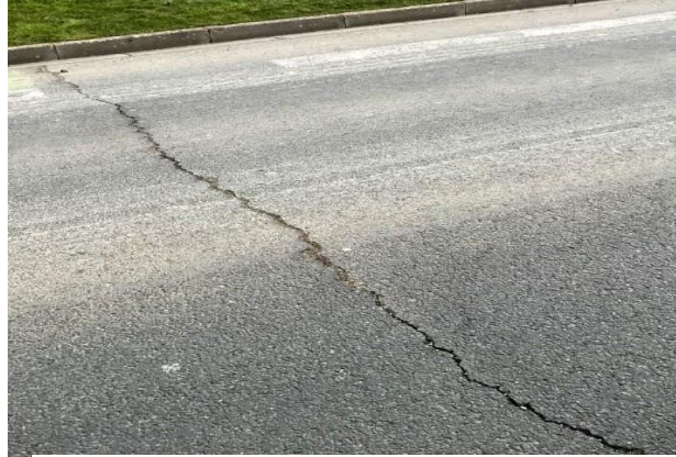
Figure I-1 : Fissure transversale.
