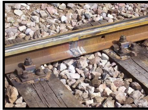
Figure 9 : Long rail soudé (LRS)
