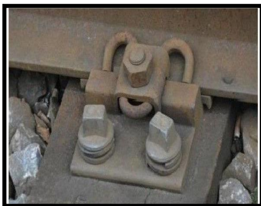
Figure 1 Attache de type E-clip
