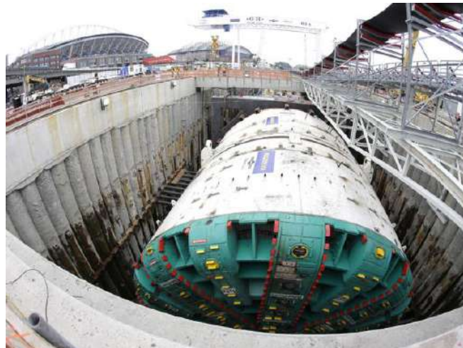
Figure I.11 Tunnelier
