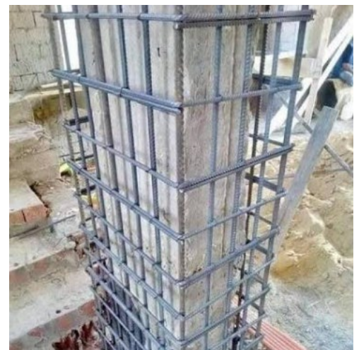
Figure 62: Chemisage des poteaux
