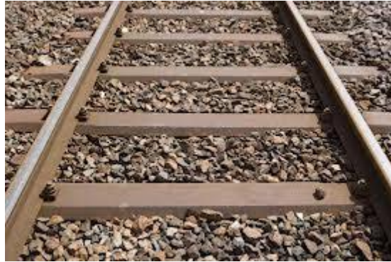
Figure III.5 Traverse métallique
