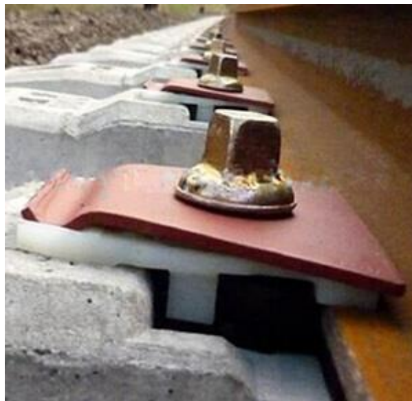
Figure III. 6 Attache type Nabla
