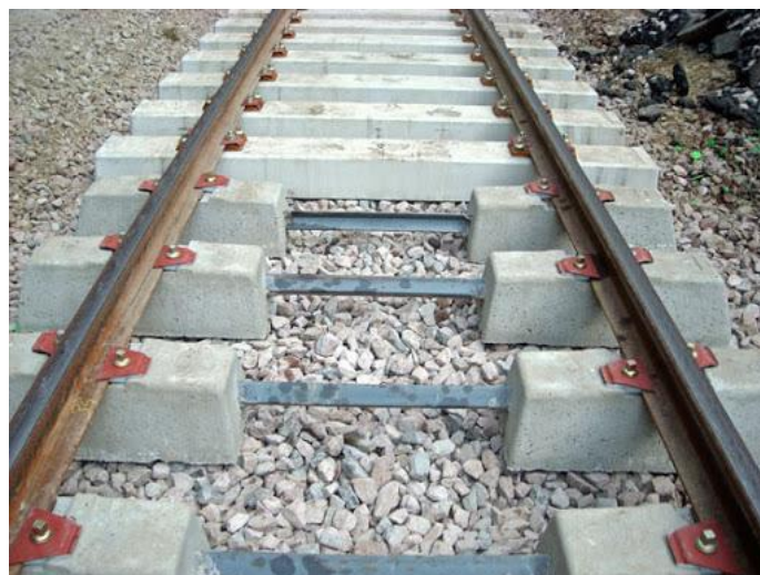
Figure III.4 Traverse en BA
