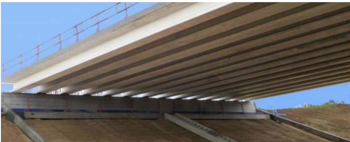
Figure I.03 Pont a poutres
