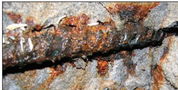
Figure I.12 Armature corrodée
