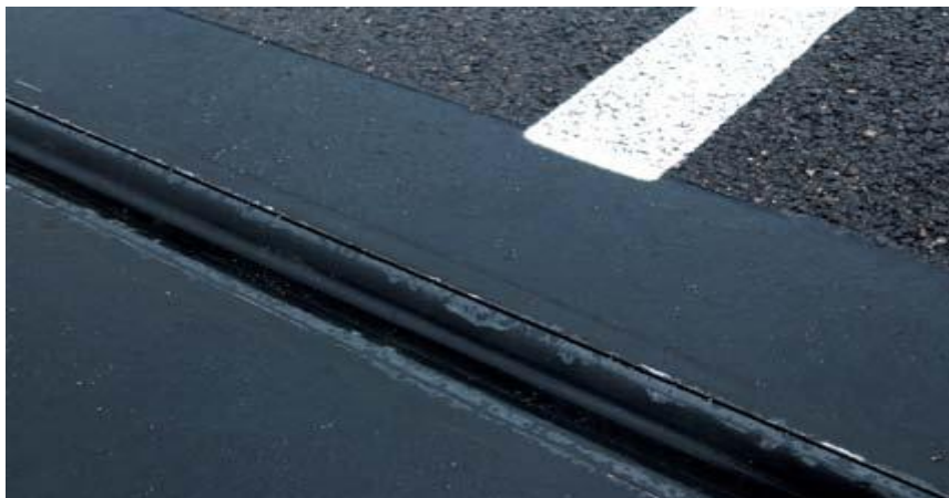
Figure VII.1 Joint de chaussée JEP3
