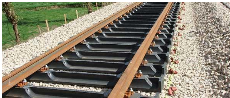
Figure II-6: Traverse en acier
