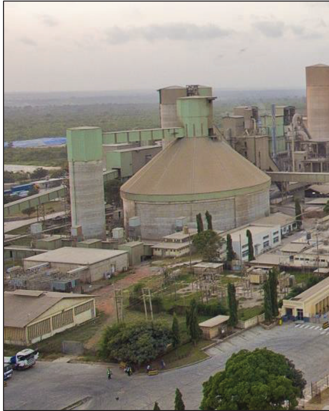
Figure II-10 : silo clinker - Dar Es Salaam, Tanzanie [12]
