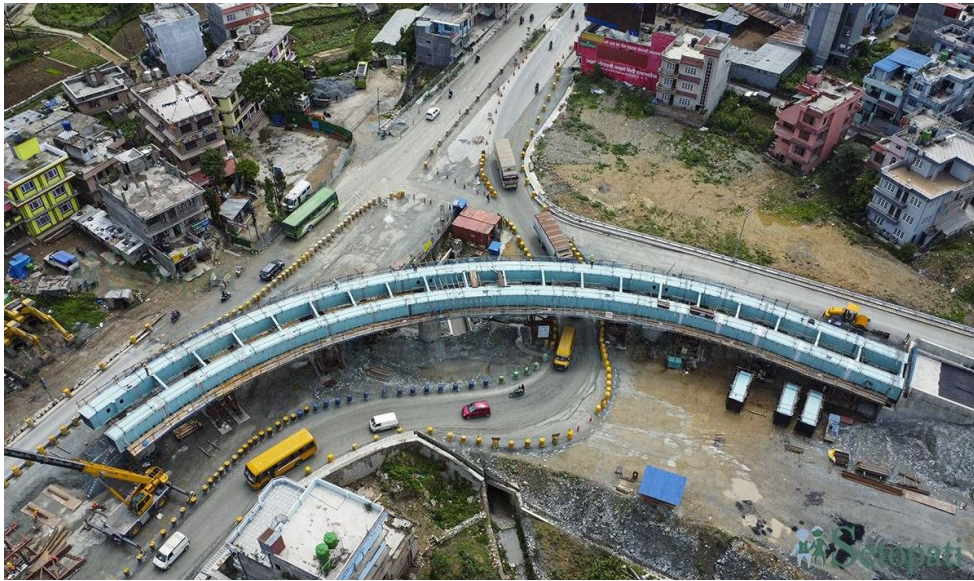
Figure III.3. Balambu Steel Box Bridge, Nepal.
