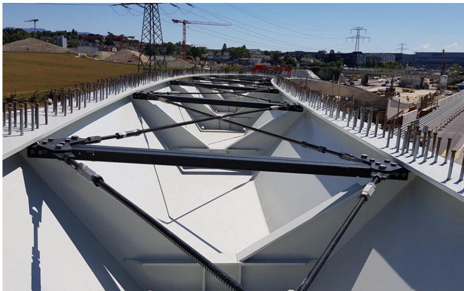
Figure III.4. Steel box girder example.
