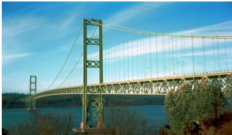
Figure I.5. The Tacoma Bridge after renovation.
