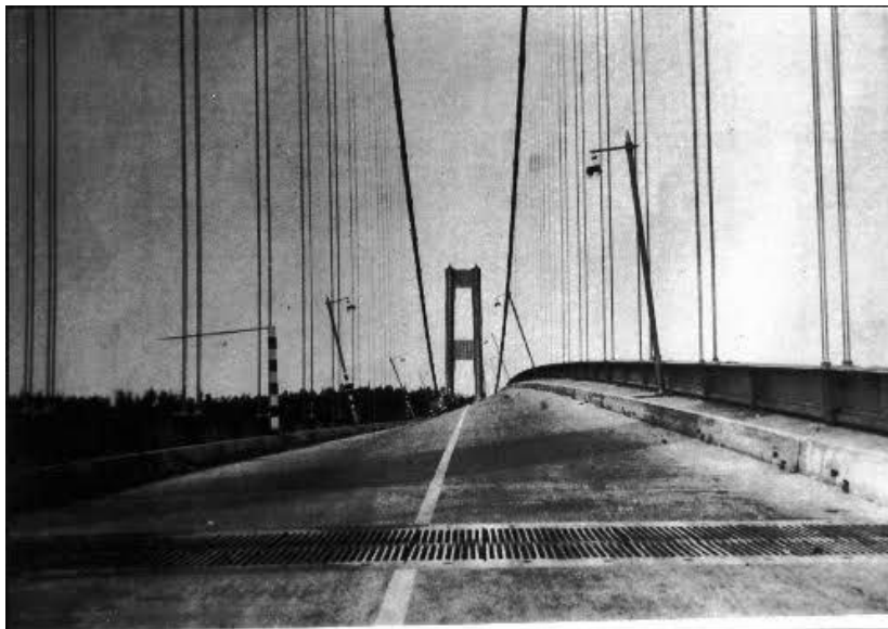
Figure I.2. Tacoma Bridge Torsion Mode.
