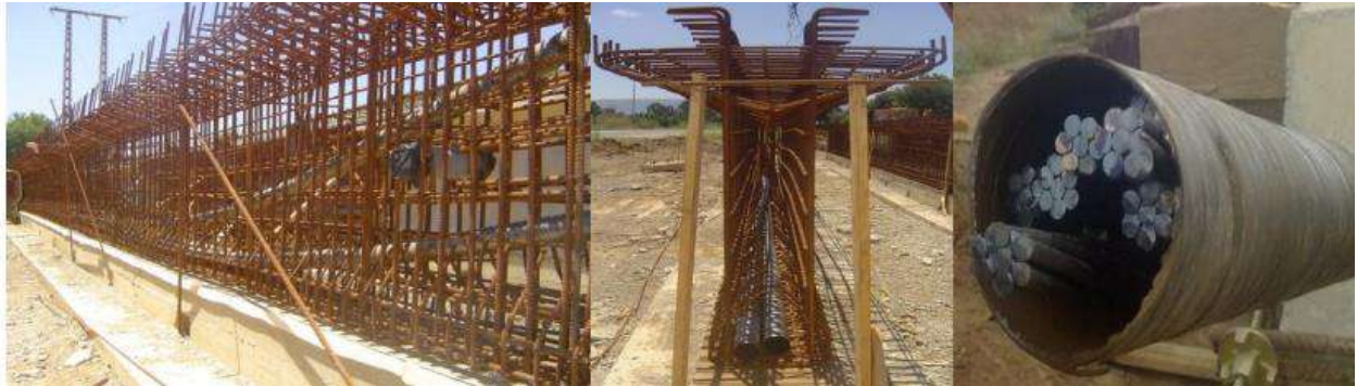
Figure XIII.13 : armatures passives et active
